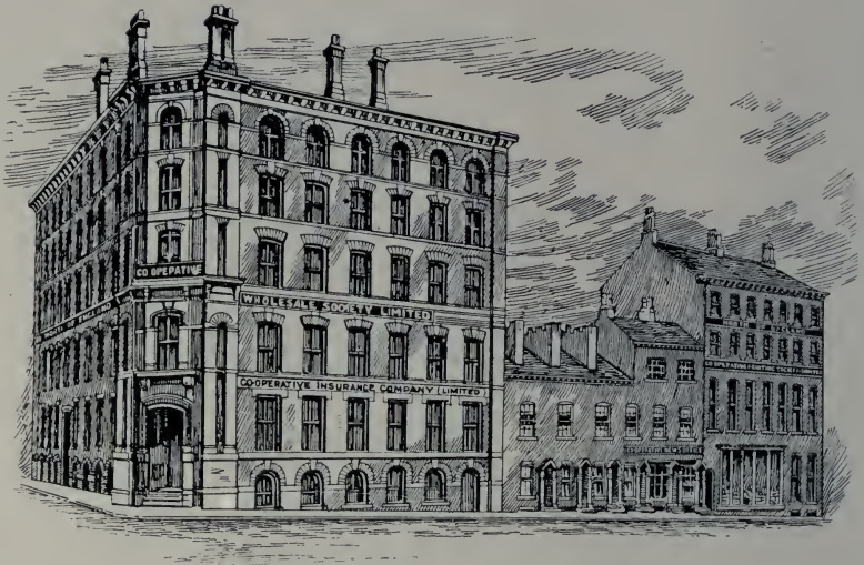
Original Balloon Street Premises.
