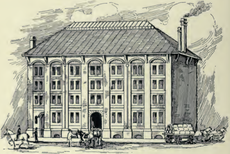
Newcastle Branch, Waterloo Street, in 1876.
