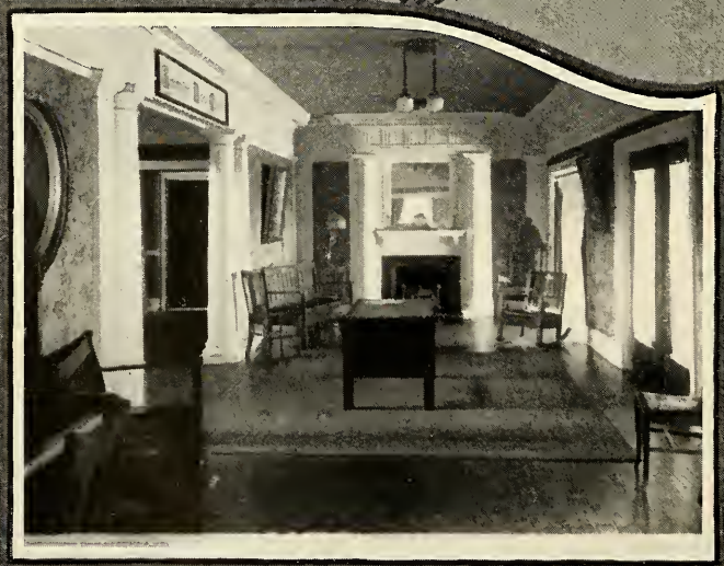
Two Views of Entrance Corridor
