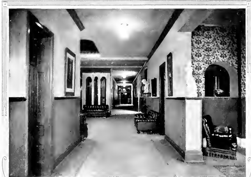
In the Main Corridor of the Girls' Dormitory
