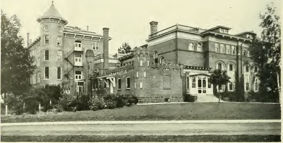
Partial View of Annex
