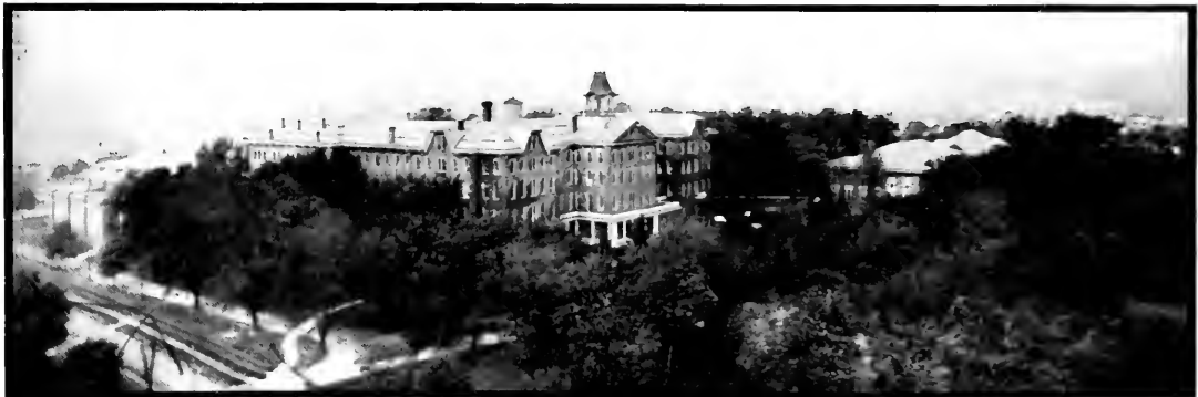
View of Campus from Top of Power House Chimney
