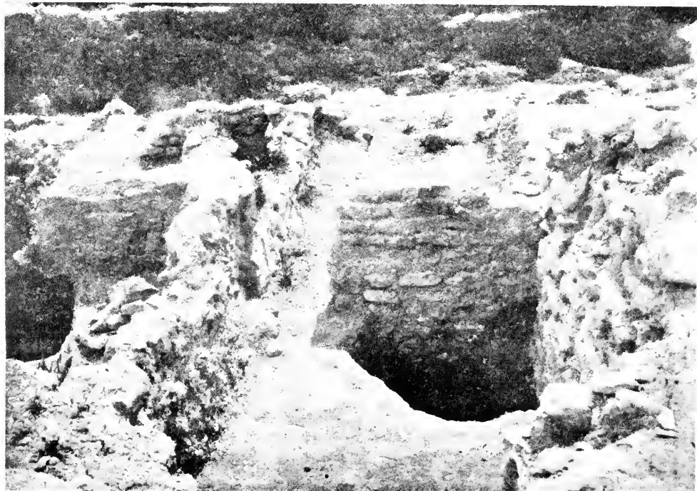
FIG. 1.—UPPER PART OF WALLS OF MAGAZINES IN N.E. QUARTER OF PALACE, SHOWING BRICK COURSES ABOVE RUBBLE MASONRY.
