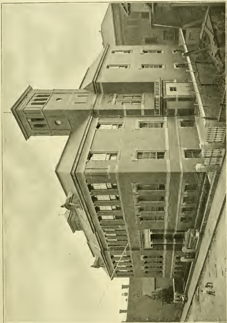
WESTON STREET SCHOOL.
