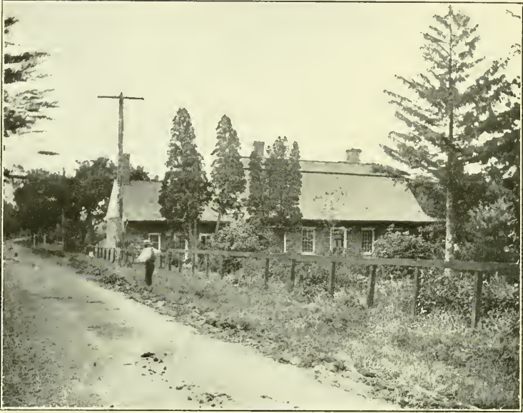
OLD BRINKERHOFF HOUSE
