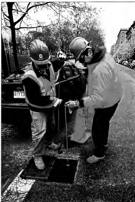
Installing a data-logger
