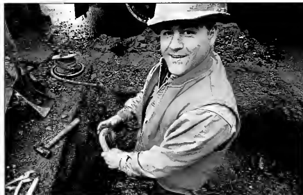
Repairing the infrastructure
