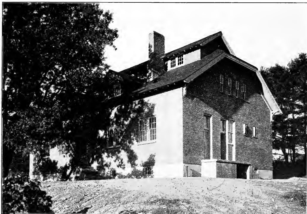
Fruit Storage Building and Laboratory, erected in 1910-11.
