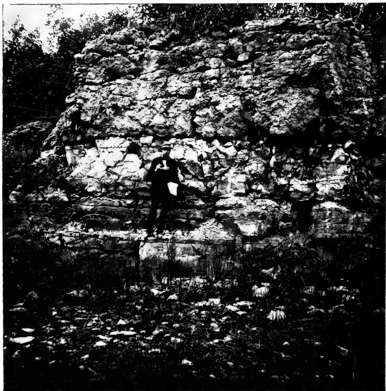
In Britton's limestone quarry 3 miles south of Syracuse. The part above the man's head is the Stromatopora limestone (Helderbergian (?)). The lower layers are the Manlius waterlime, the middle layer a compact blue limestone.
