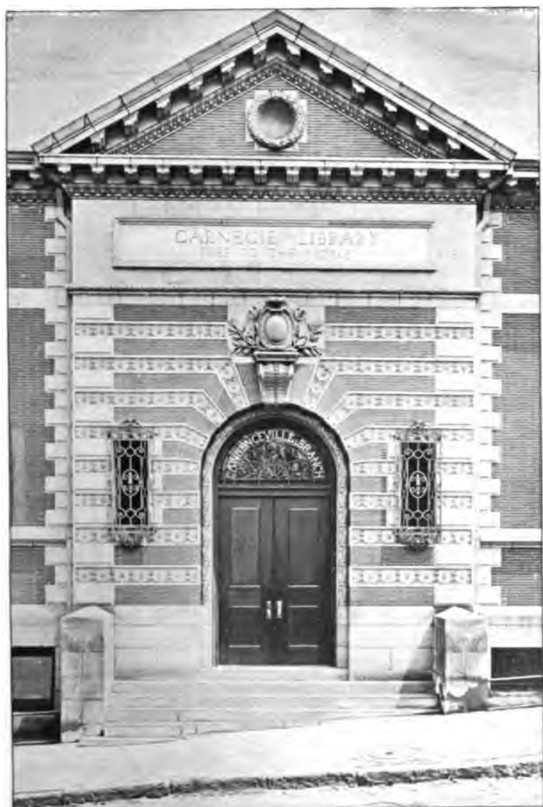
LAWRENCEVILLE BRANCH--DETAIL OF ENTRANCE.
