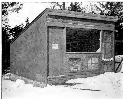
A cheap and very satisfactory type of hen house. It is neat and warm and gives opportunity for fresh air for the birds
