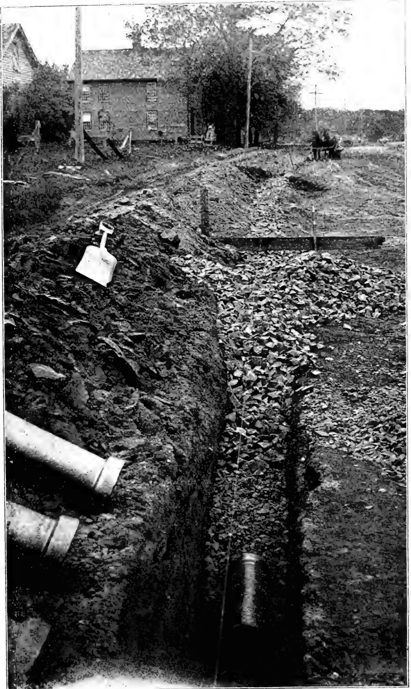
WESTFIELD ROAD, MASS., 1894. View showing details of drain.
