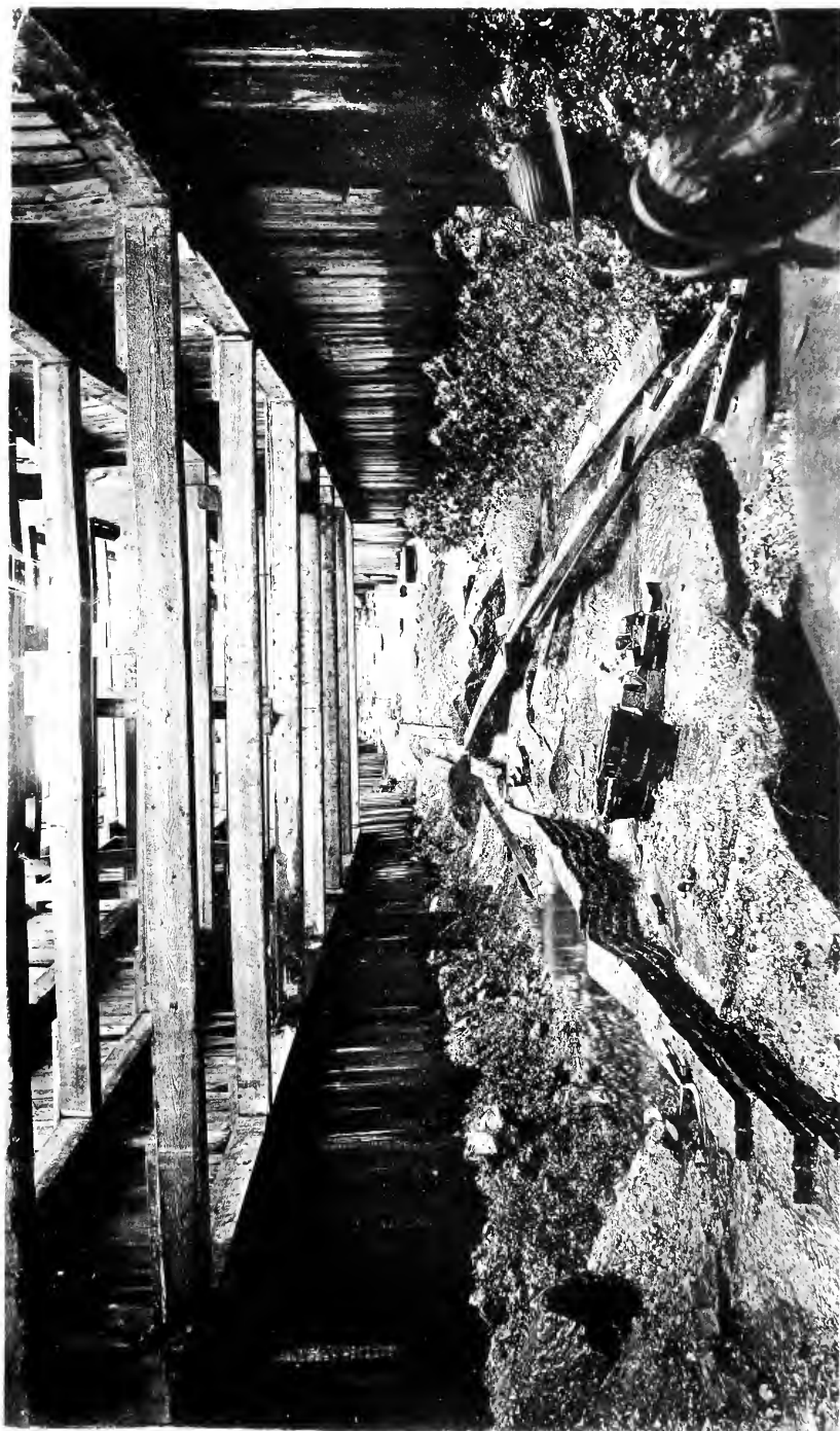
DAM NO. 5.—VIEW OF BOTTOM OF TRENCH OF CORE WALL.
