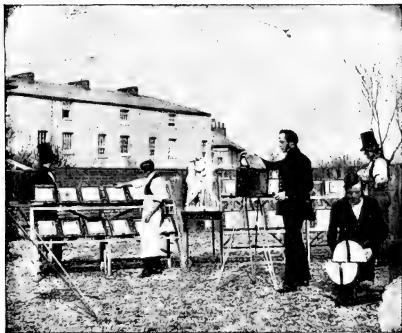
FIG. 2.—CALOTYPE PRINTING OUTFIT. From "Photominiature."
