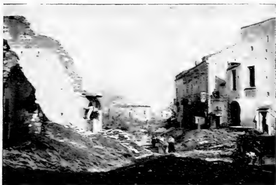
RUINED HOUSES AT OTTAVIANO.
