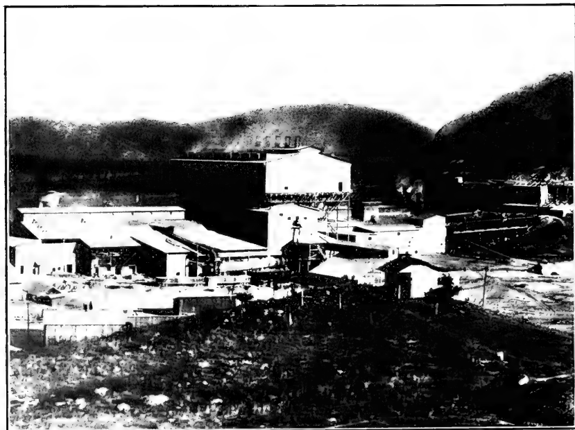
FIG. 53.—RIVERSIDE PORTLAND CEMENT WORKS AFTER INSTALLATION OF PERMANENT ELECTRIC PRECIPITATION EQUIPMENT.
