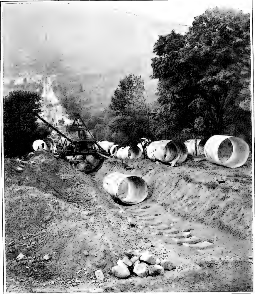
PLACING THE 9½ FOOT STEEL PIPES—FOUNDRY BROOK SIPHON.
