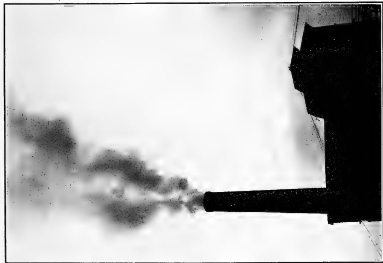
FIG. 30.—MAIN STACK, BALAKALA SMELTER, ELECTRIC CURRENT OFF.
