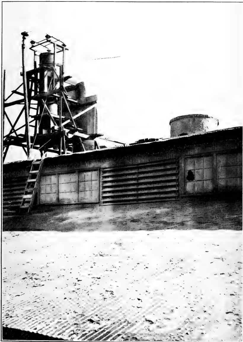
FIG. 49.—EARLY EXPERIMENTAL PRECIPITATOR AT RIVERSIDE PORTLAND CEMENT WORKS.
