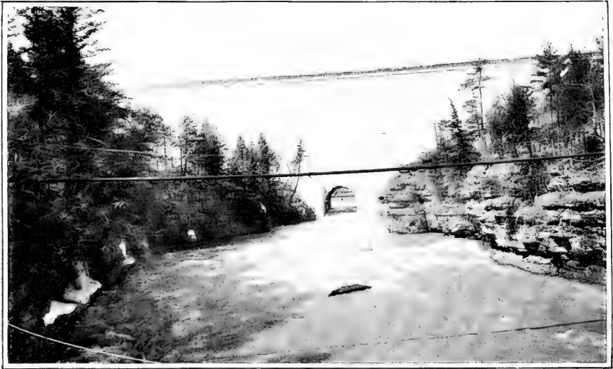
OLIVE BRIDGE DAM. ESOPUS CREEK FLOWING THROUGH TEMPORARY TUNNEL.
