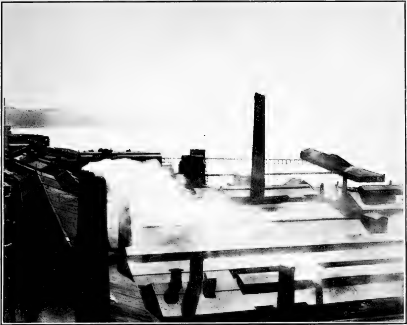
FIG. 11.—PARTING-ROOM STACK, SELBY SMELTER, ELECTRIC CURRENT OFF.
