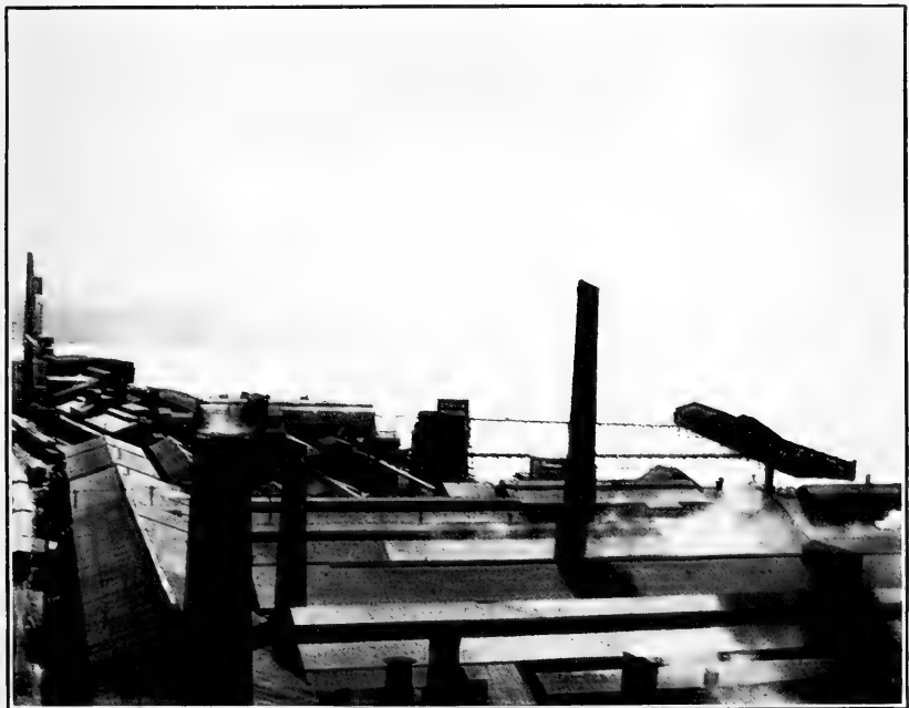
FIG. 12.—PARTING-ROOM STACK, SELBY SMELTER, ELECTRIC CURRENT ON.
