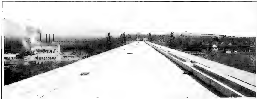
DRIVEWAY ALONG CREST OF OLIVE BRIDGE DAM. This will form part of a system of new highways.
