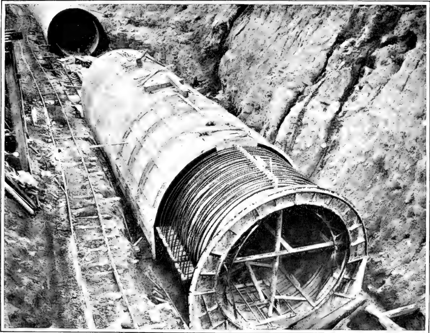
CONSTRUCTING A STEEL AND CONCRETE SECTION OF AQUEDUCT.
