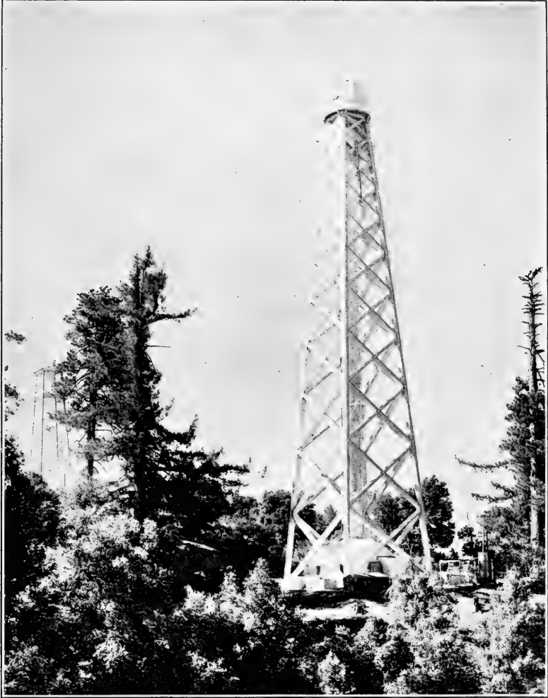
FIG. 12.—150-FOOT TOWER TELESCOPE.
