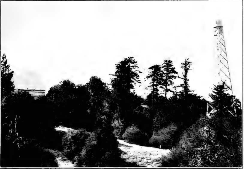
1. CARNEGIE SOLAR OBSERVATORY, MOUNT WILSON, CALIF. 160-FOOT TOWER AND 60-INCH DOME.
