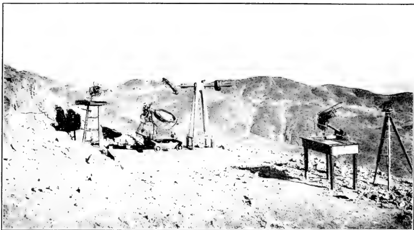
1. MONTEZUMA SOLAR OBSERVING STATION, CHILE. COELOSTAT AND PYRHELIOMETRIC APPARATUS.
