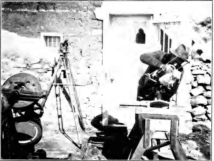
2. COELOSTAT AND PYRHELIOMETER, MOUNT HARQUA HALA.
