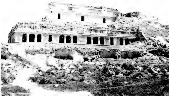
2. A palace-type structure of the Mayan ceremonial center of Sayil, Yucatan, Mexico. This handsome building, now largely in ruins, was built of rubble faced with cut limestone blocks and mortar. It is estimated to have contained about 100 rooms. It was probably constructed, at least in its final phases, between A.D. 600 and 900.
