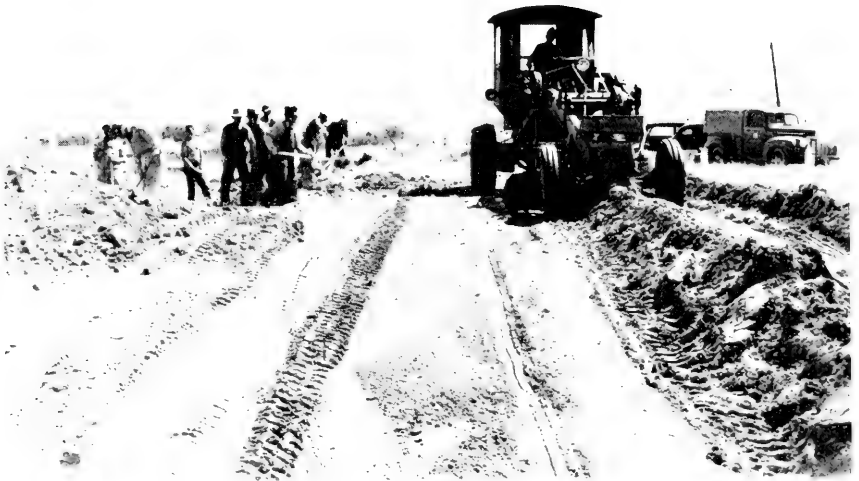
1. Using road-building equipment to clear overburden from village site.
