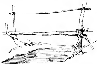
FIG. 334.—An Indian bridge with hand rail on the upper Rupununi River.
