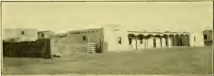
b. HOUSES ON EAST SIDE OF PLAZA
