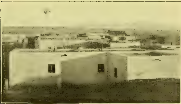
c. SOUTHEAST PART OF TOWN. MANZANO MOUNTAINS IN BACKGROUND
