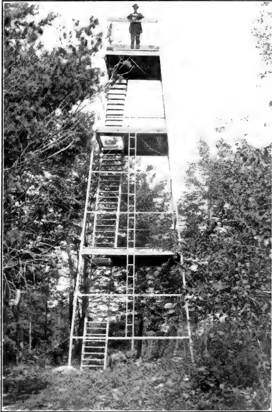
Steel tower (45 feet high) on Twadell Point Observ- vation Station, East Branch, N. Y.
