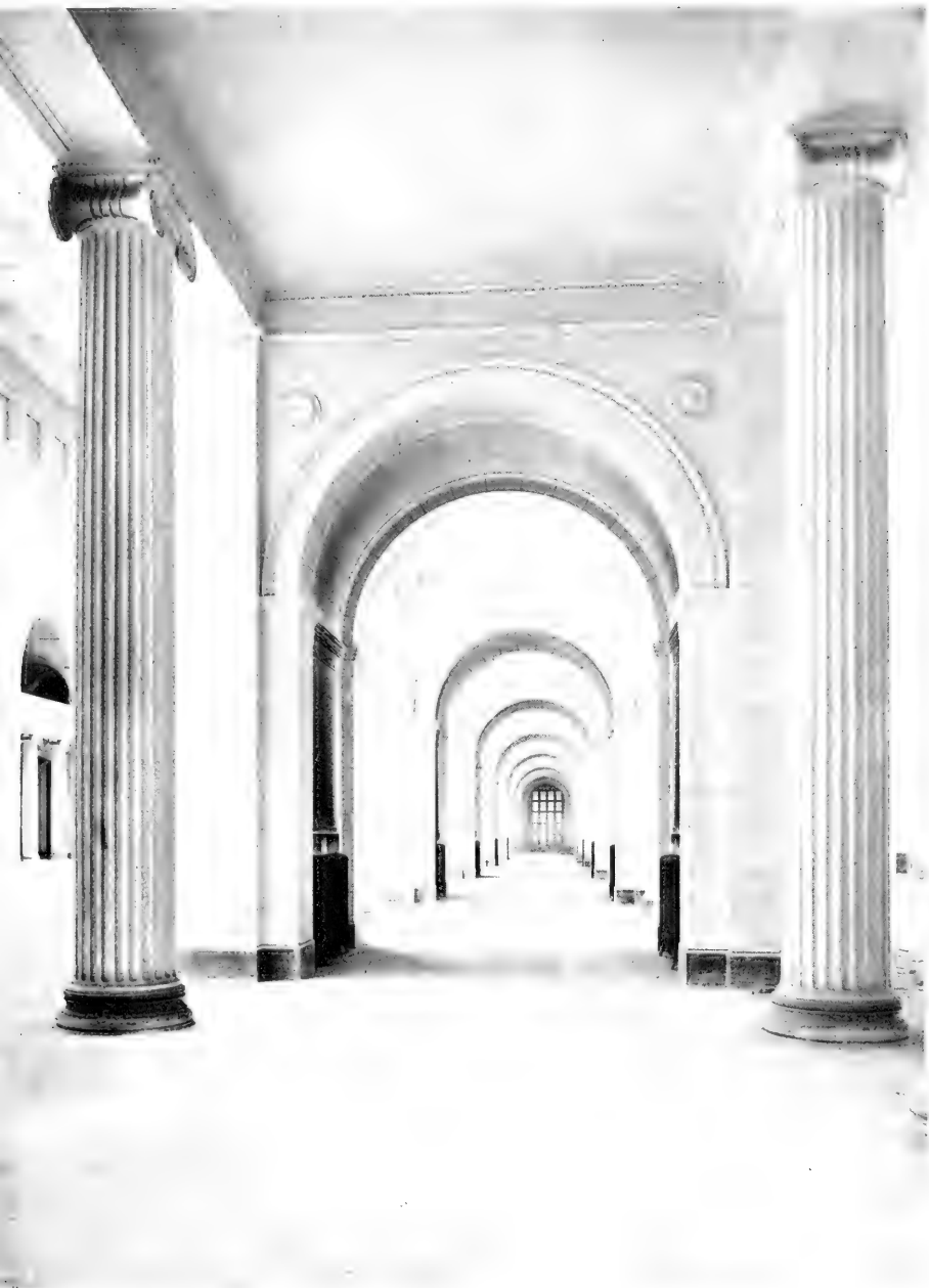
WEST COLONNADE PARALLELING STANLEY FIELD HALL, FIRST FLOOR LOOKING SOUTH.
