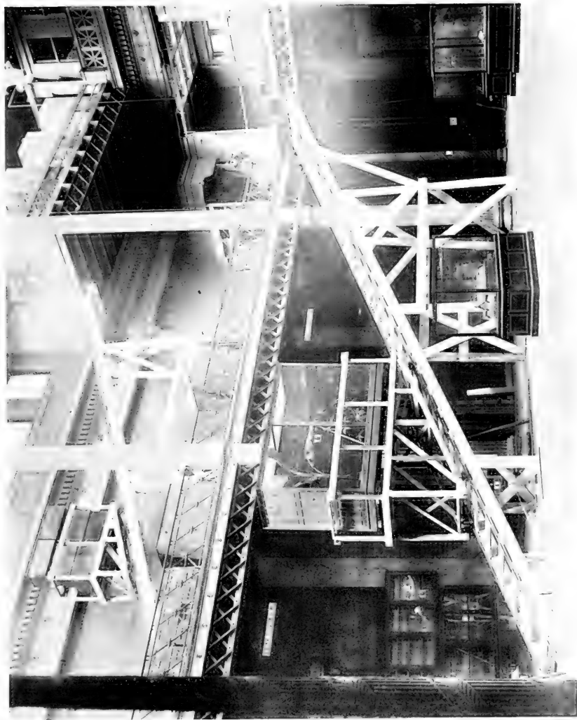
GRAVITY TRAMWAY FROM UPPER GALLERIES TO MAIN FLOOR, OLD BUILDING. Lower car conveying twelve-foot exhibition case with installation intact.
