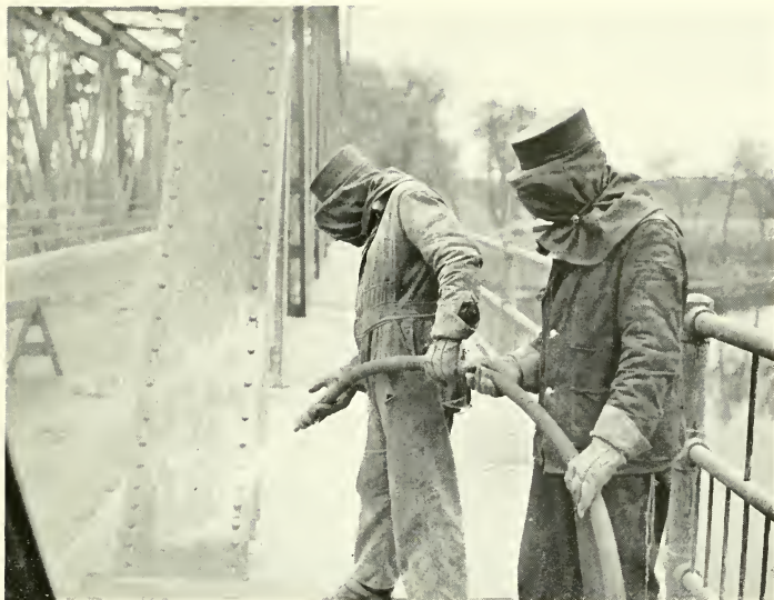
Painting is a necessary part of the City's bridge maintenance activities. Wearing protective masks workmen are shown sandblasting a bridge in preparation for painting
