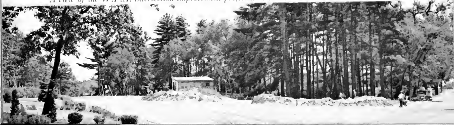
A view of the W.P.A. intersection improvement project at Carter, Bow and South Streets
