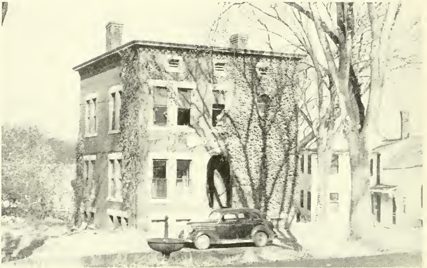
This building at Penacook, formerly occupied as a police station, will be converted into a modern branch library
