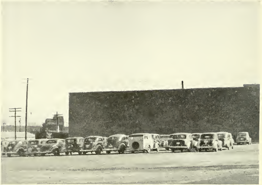
Traffic congestion on upper Main Street was greatly relieved by this new off-street parking lot at the Rumford Press
