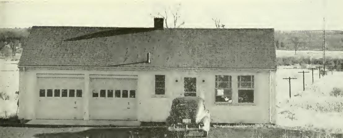
Transmitting facilities of radio station WKXL
