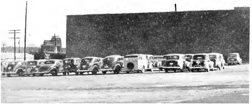
Traffic congestion on upper Main Street was greatly relieved by this new off-street parking lot at the Rumford Press
