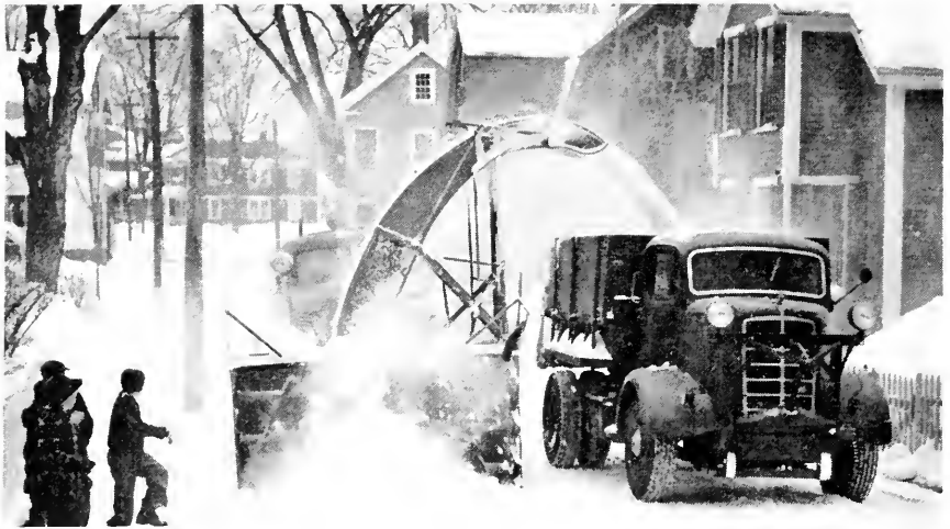
Public Works Sno-Go helped remove 128,000 cubic yards of snow from City roads during 1948.
