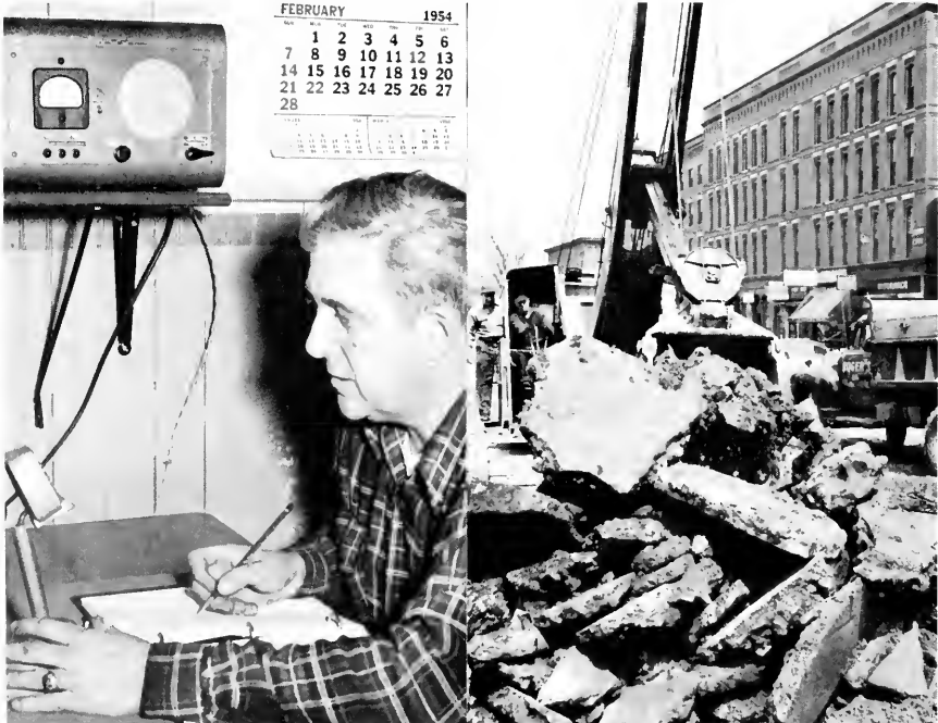
(Right) A steam shovel aids in rebuilding Main Street.
