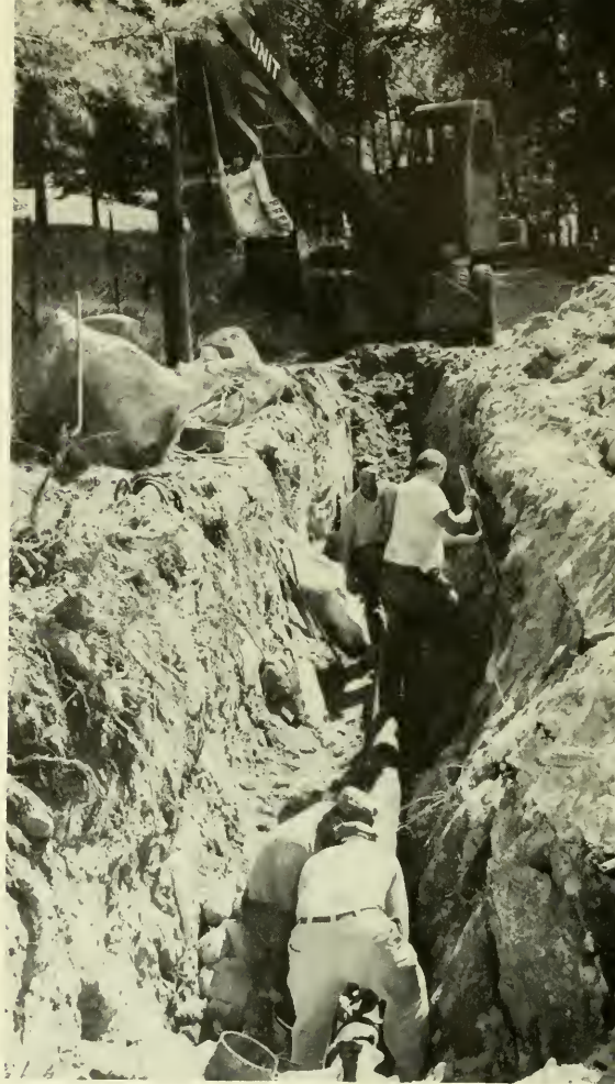
Water Department crew lays new main in River Road, Penacook.
