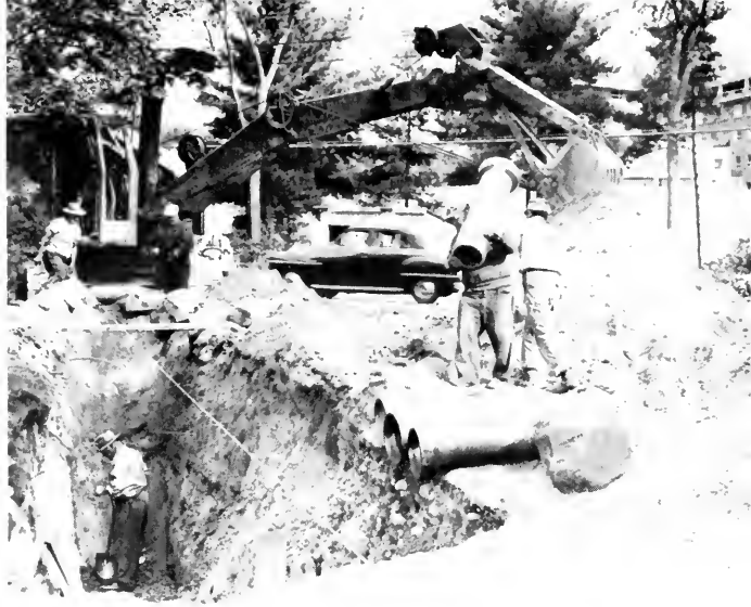
Laying the sewer in Pleasant Street near the new Concord Hospital
