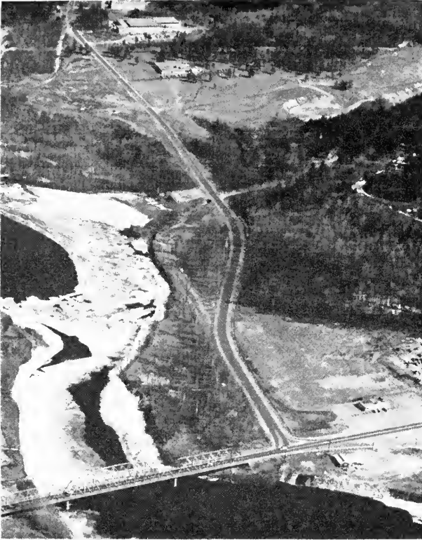
This photo indicates 0.3 of a mile on realignment of Old Turnpike Road traveling east from Manchester Street to one of Concord's newly developing industrial centers. Total cost for this project was $23,200.00.
