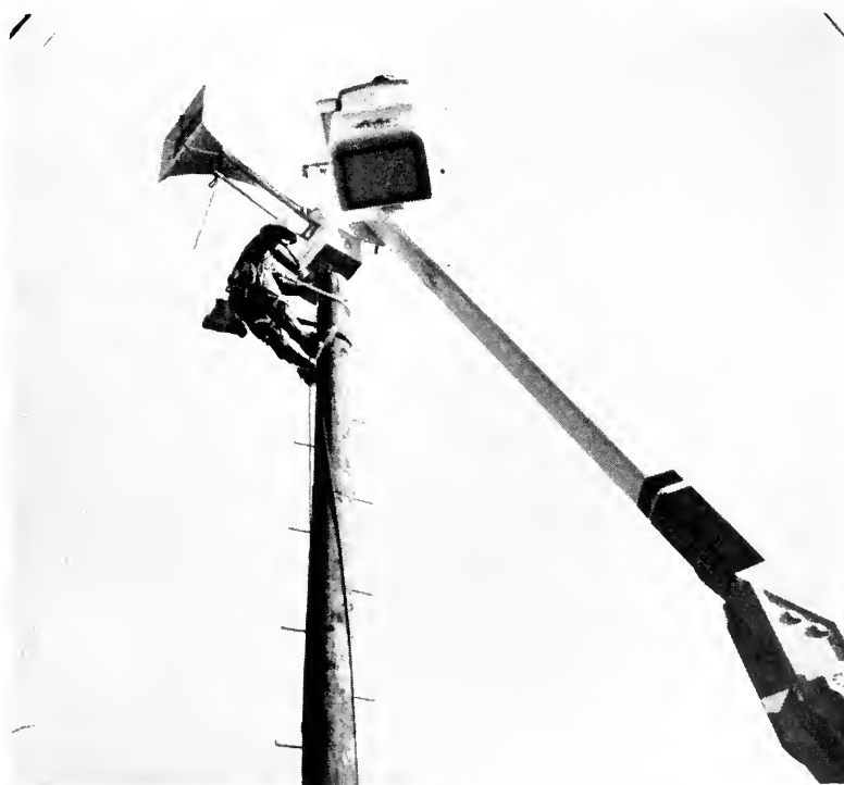
One of five air raid sirens being installed in city. Electric Company bucket truck was used to raise siren more than forty feet in the air.
