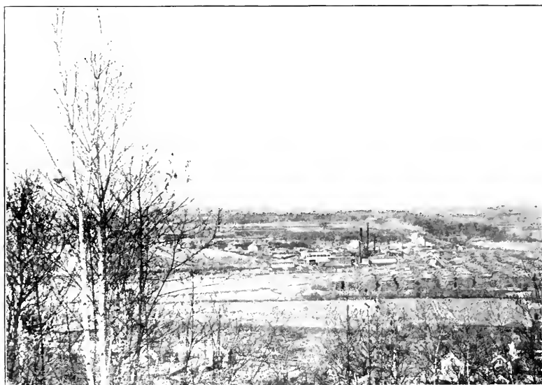
Connecticut River Lumber Company, Mount Tom Junction, Massachusetts. The largest sawmill in the State.
