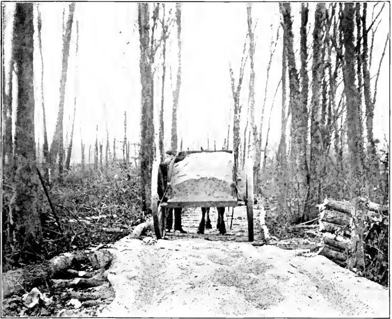
Stevens estate, North Andover. Putting sawdust on corduroy road used in logging.
