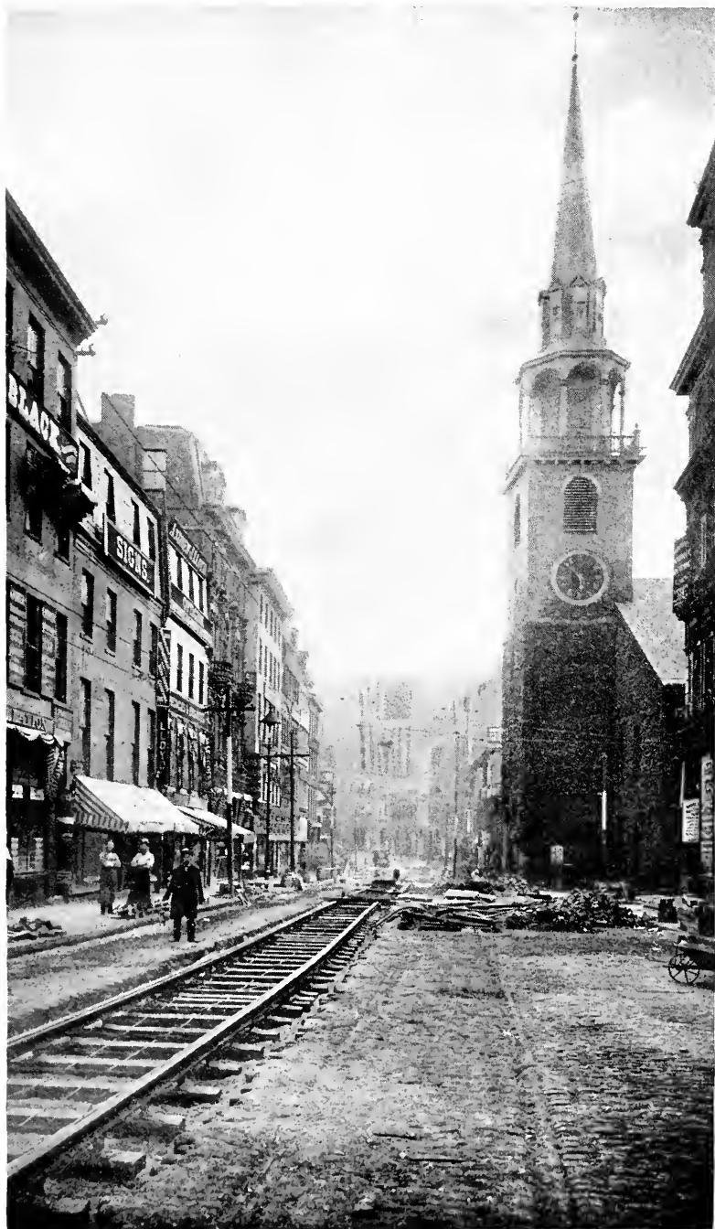
TRACK CONSTRUCTION, WASHINGTON STREET.
