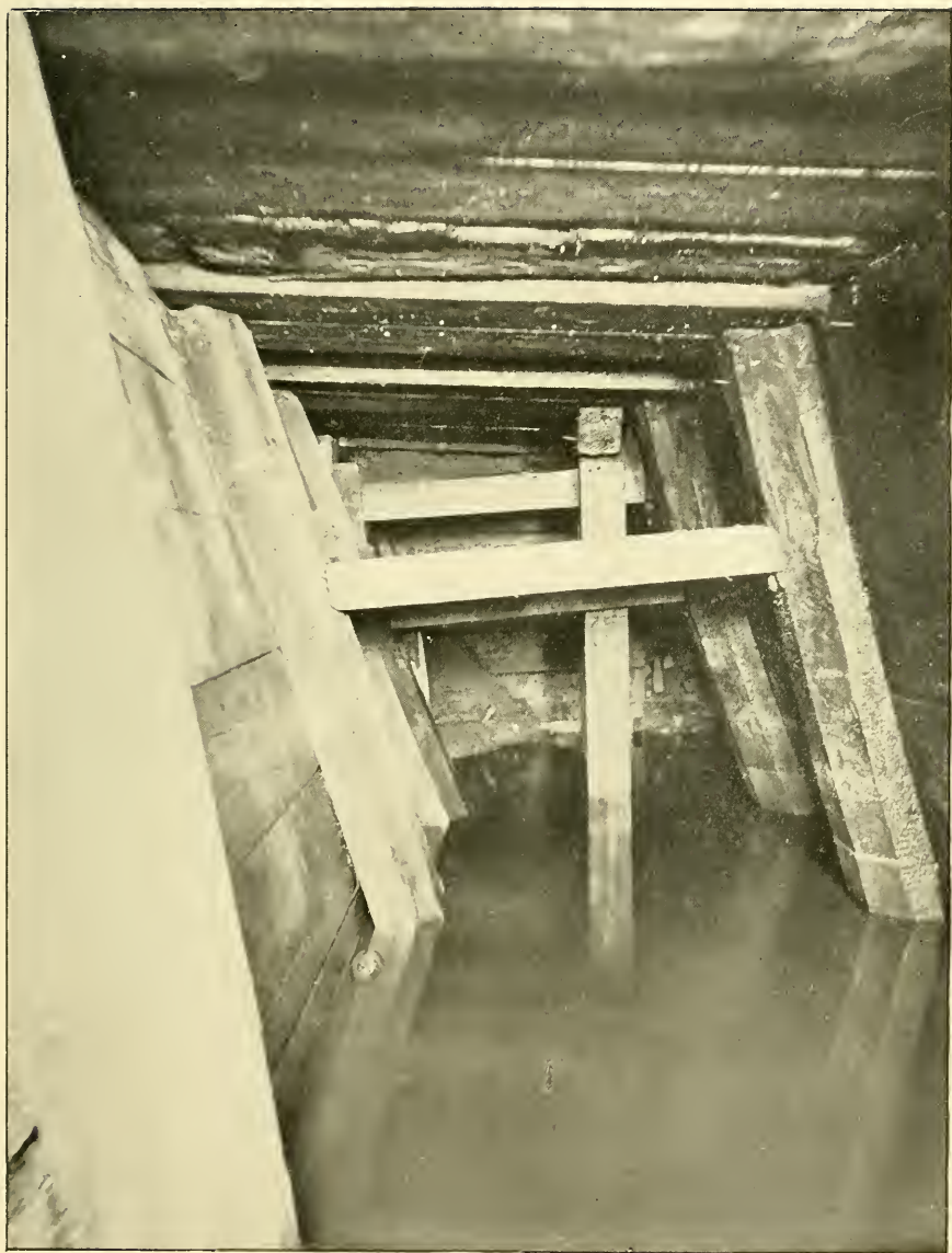
OLD WOODEN SEWER—DOVER STREET.
