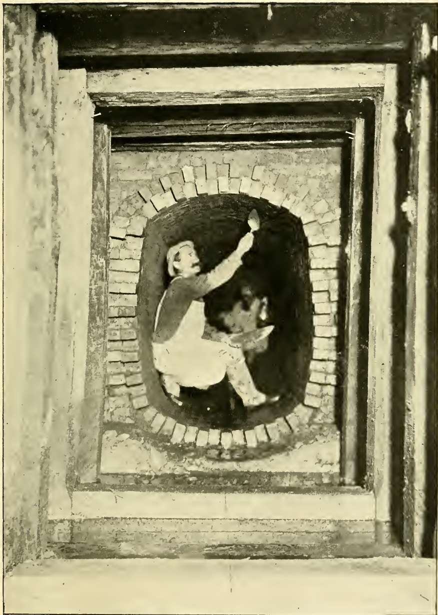
MASONRY CONSTRUCTION WITHIN DOVER-STREET SEWER.
