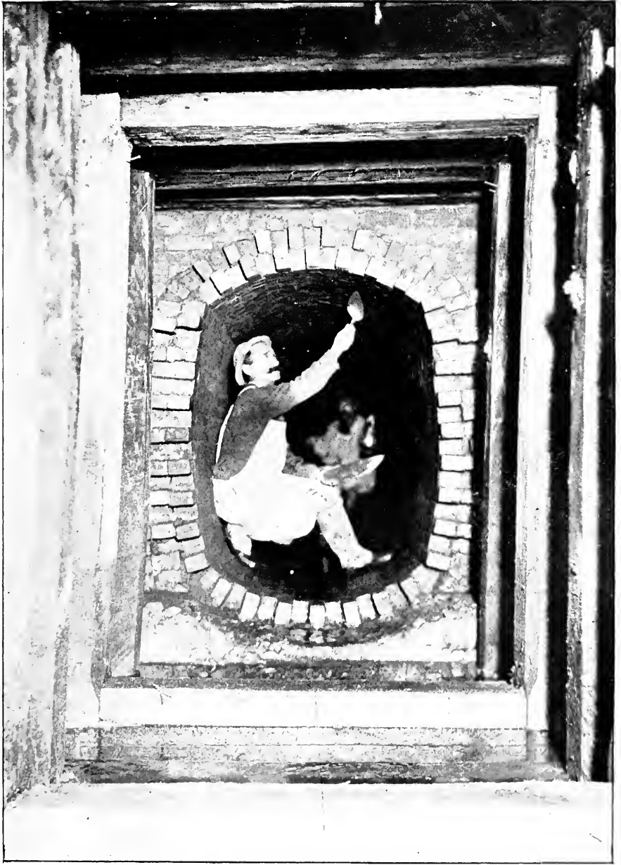
MASONRY CONSTRUCTION WITHIN DOVER-STREET SEWER.
