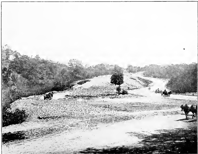
COMMONWEALTH AVENUE, NORTH OF WALLINGFORD ROAD.
