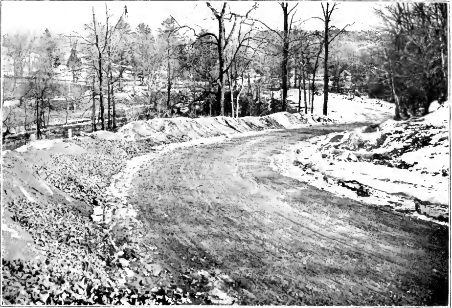
VIEW OF LAKE FANNIE HILL, SHOWING BANK CONSTRUCTED ON LEFT TO PREVENT ACCIDENTS.
