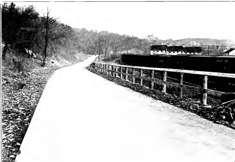
VIEW OF CONCRETE ROAD BETWEEN WEVERTON AND KNOXVILLE, IN FREDERICK COUNTY, THE FINAL LINK IN THE STATE ROAD SYSTEM BETWEEN BALTIMORE AND HARPER'S FERRY, W. VA.
