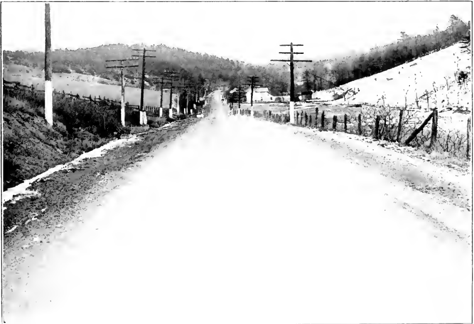
VIEW OF GENERAL MAINTENANCE ON BALTIMORE PIKE, IN ALLEGANY COUNTY, EAST OF CUMBERLAND.
