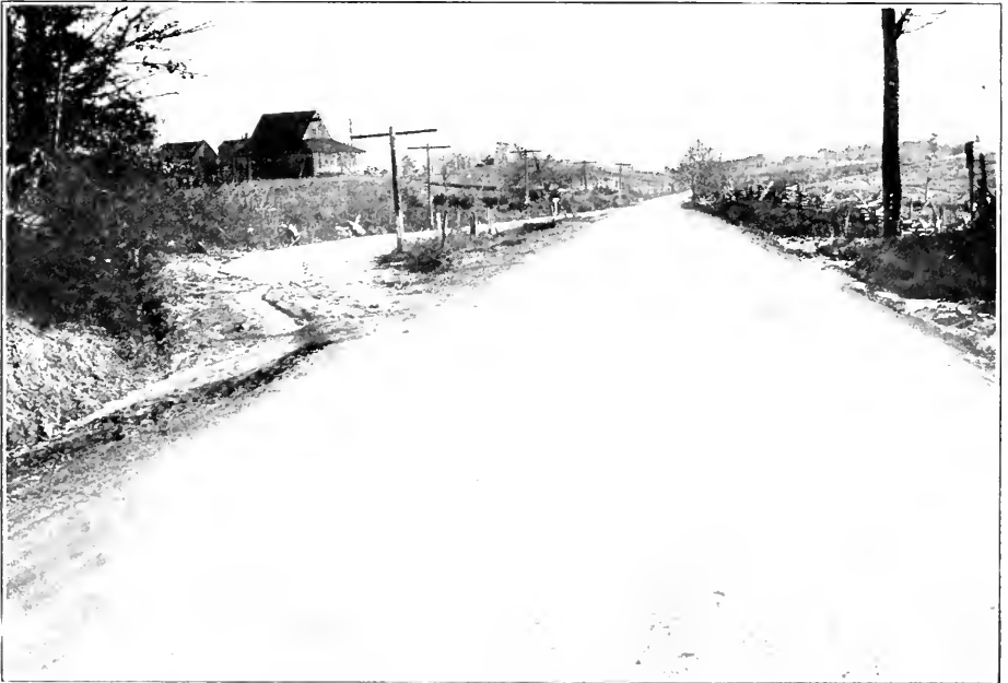
VIEW SHOWING RELOCATION OF GRAVEL ROAD ON THE OWINGS SOLOMON'S ISLAND ROAD, IN CALVERT COUNTY, TO IMPROVE ALIGNMENT.
