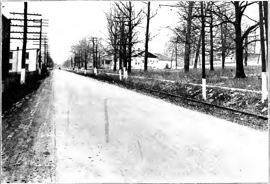
VIEW OF CONCRETE ROAD ON THE NATIONAL PIKE, THROUGH LA VALE, ALLEGANY COUNTY.
