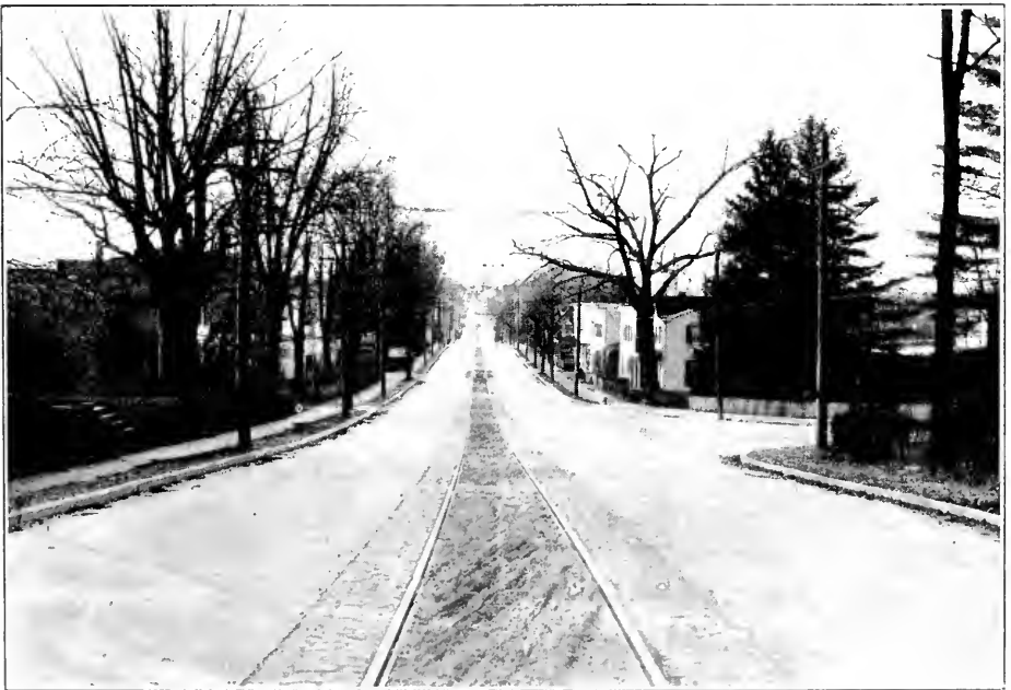
GENERAL VIEW OF MAIN STREET, ROCKVILLE, SHOWING CONCRETE STREET, WITH CURB AND GUTTER ON EACH SIDE.
