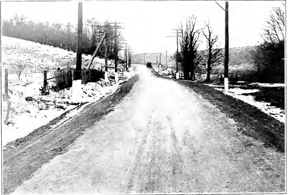
VIEW OF GENERAL MAINTENANCE ON FREDERICK ROAD, IN HOWARD COUNTY
