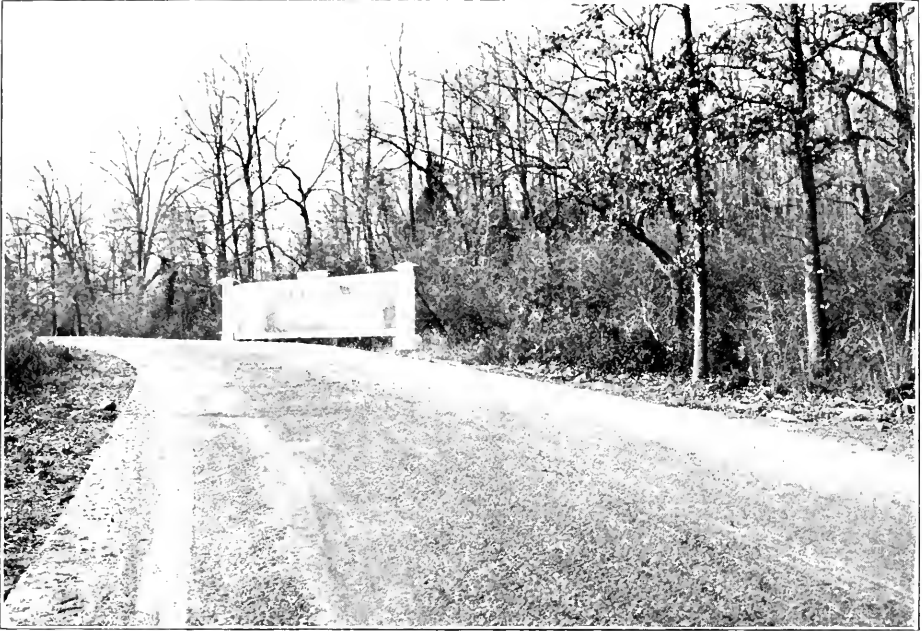
VIEW OF BELAIR ROAD IN BALTIMORE COUNTY, SHOWING CONCRETE SHOULDERS AND BANKED CURVE.
