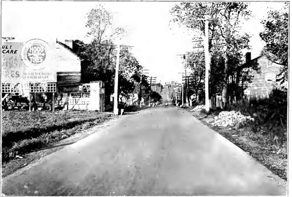
FINISHED SHEET ASPHALT PAVEMENT ON THE BALTIMORE AND WASHINGTON BOULEVARD, IN BALTIMORE COUNTY.
