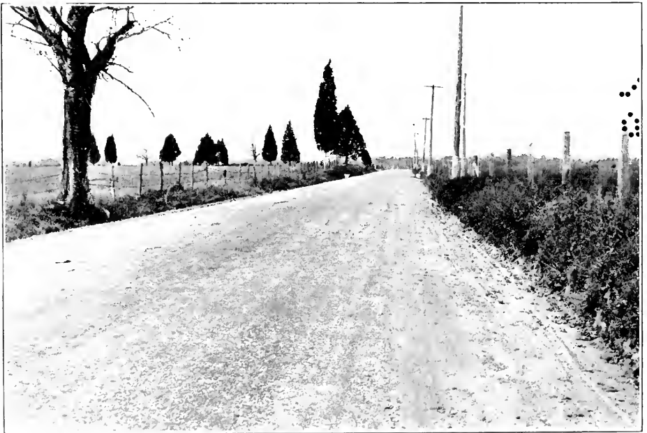
GENERAL VIEW SHOWING MAINTENANCE OF MACADAM ROAD IN TALBOT COUNTY, BETWEEN EASTON AND WYE MILLS
