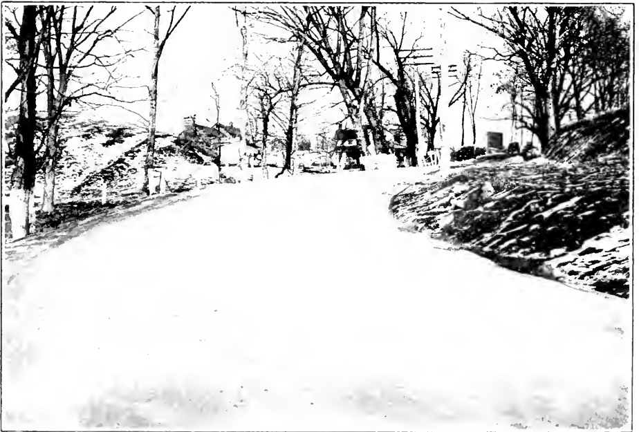
VIEW SHOWING BANK ON LAKE FANNIE HILL, IN HARFORD COUNTY, GRADED TO IMPROVE VISION.
