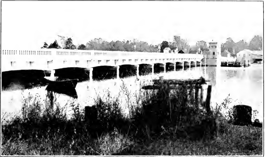
GENERAL VIEW OF SASSAFRAS RIVER BRIDGE FROM SOUTH SHORE.
