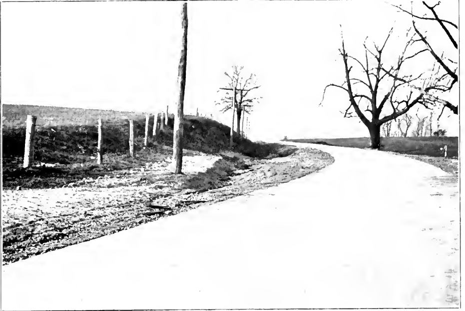
VIEW OF CONCRETE ROADWAY ON HANOVER PIKE, IN BALTIMORE COUNTY, NORTH OF GLEN MORRIS.
