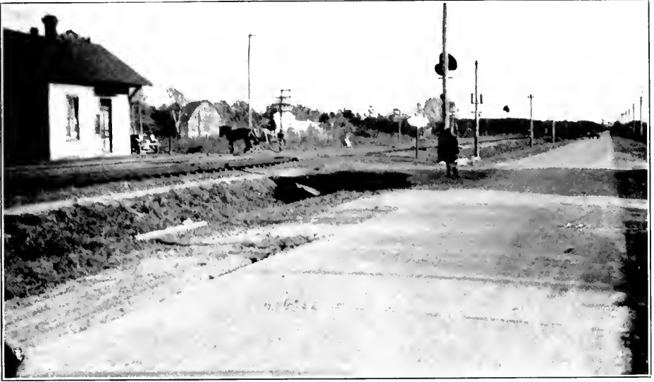
GENERAL VIEW OF BITUMINOUS CONCRETE ROAD BETWEEN WESTOVER AND POCOMOKE, IN SOMERSET COUNTY.
