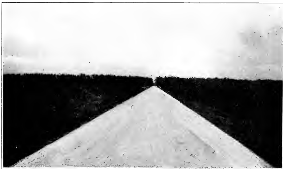
CONCRETE ROAD IN WORCESTER COUNTY, BETWEEN POCOMOKE AND THE VIRGINIA LINE.
