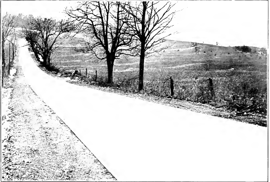
CONCRETE ROADWAY ON LITTLESTOWN TURNPIKE, IN CARROLL COUNTY.
