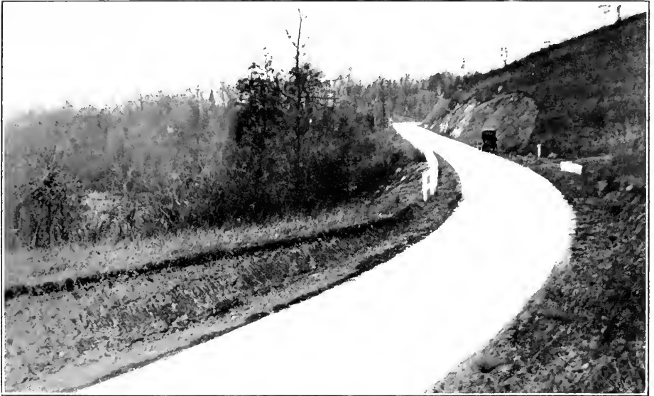
VIEW OF PORTERS BRIDGE—RISING SUN ROAD, IN CECIL COUNTY—SHOWING RELOCATION TO IMPROVED GRADE.
