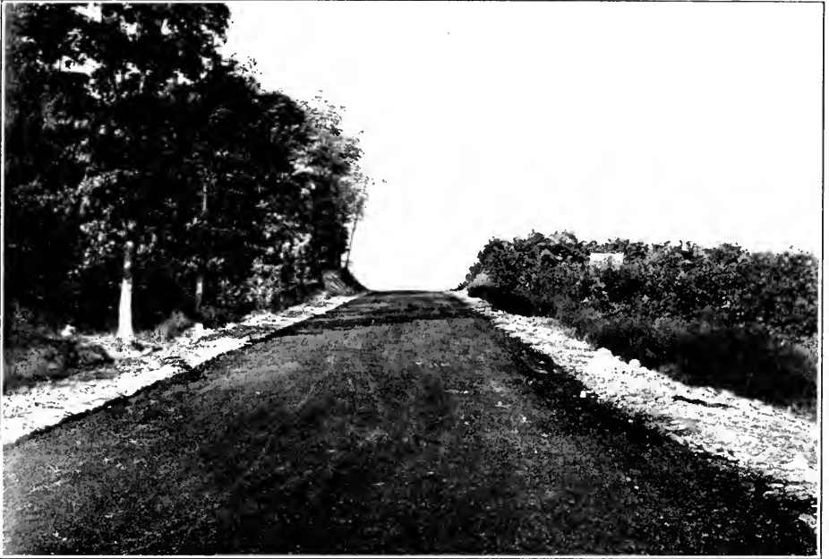
VIEW OF BALTIMORE AND WASHINGTON BOULEVARD, IN BALTIMORE COUNTY, SHOWING BINDER COURSE IN PLACE, READY TO RECEIVE ASPHALT TOPPING.
