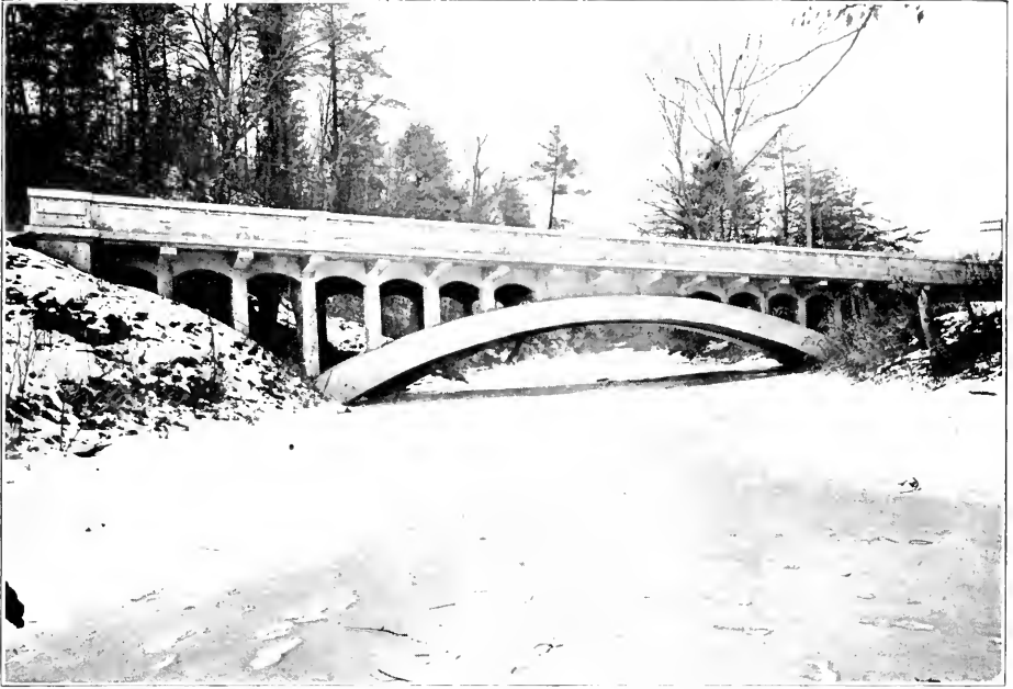
CONCRETE ARCH BRIDGE OVER FIFTEEN-MILE CREEK, IN ALLEGANY COUNTY.
