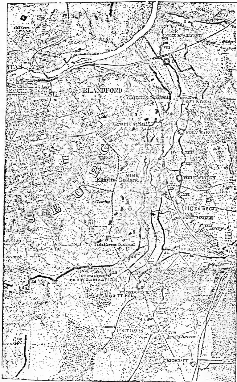
WORKS AROUND PETERSBURG, SHOWING POSITION 118TH OCCUPIED.
