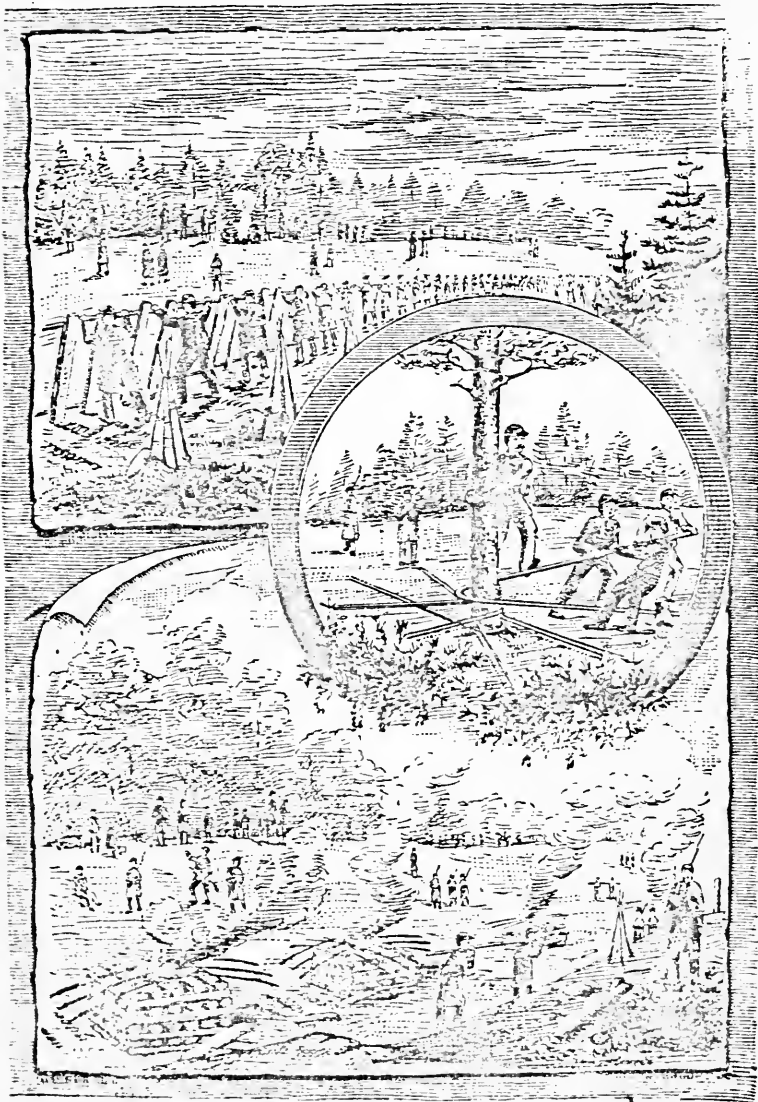
TEARING UP THE WELDON RAILROAD.
