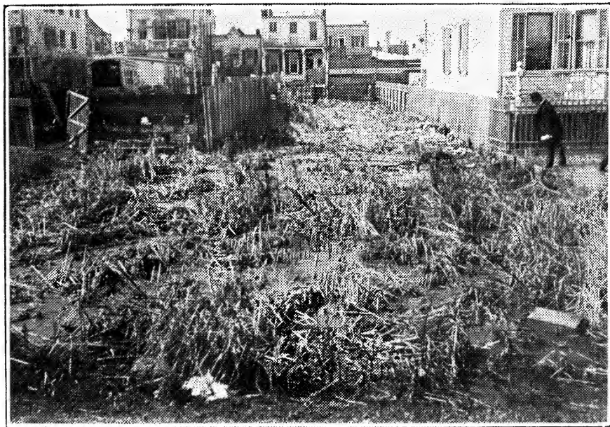
STANDING WATER ON VAN SICKLEN AVE., SOUTH OF NEPTUNE AVE., CONEY ISLAND. DWELLINGS REACHED BY BRIDGING OVER THE WET SPACES.
