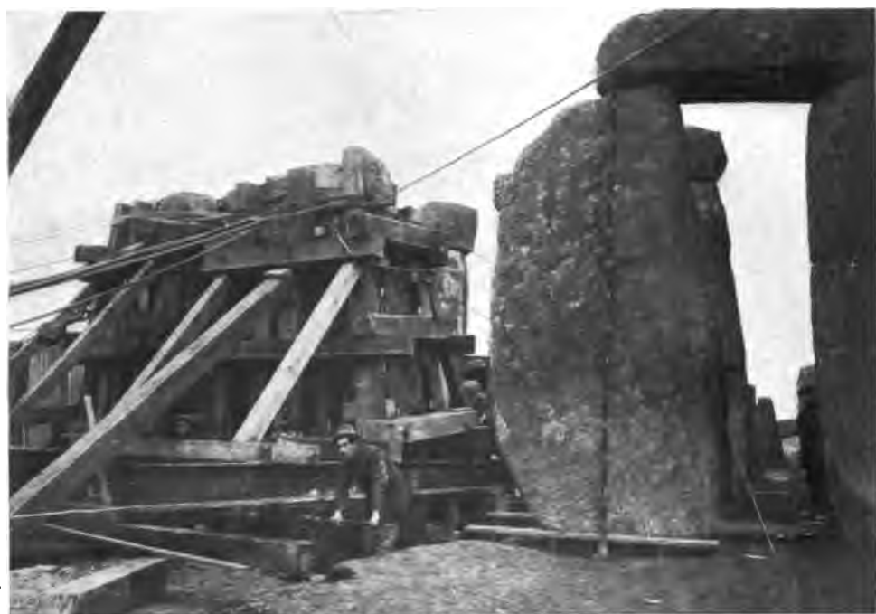
STRAIGHTENING STONE No. 6 BY MEANS OF JACKS
