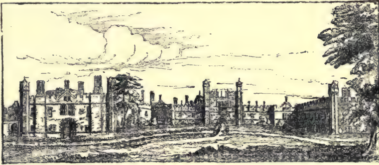
FIG. I.—WEST FRONT OF WOLSEY'S PALACE, HAMPTON COURT.
