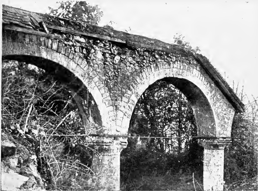
NORMAN ARCHES, HIGH WYCOMBE.
