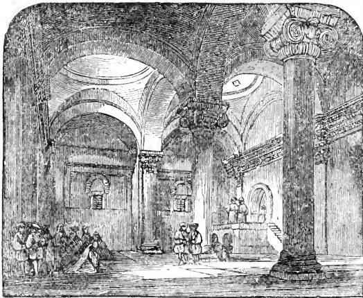
Interior view of East Gate.
