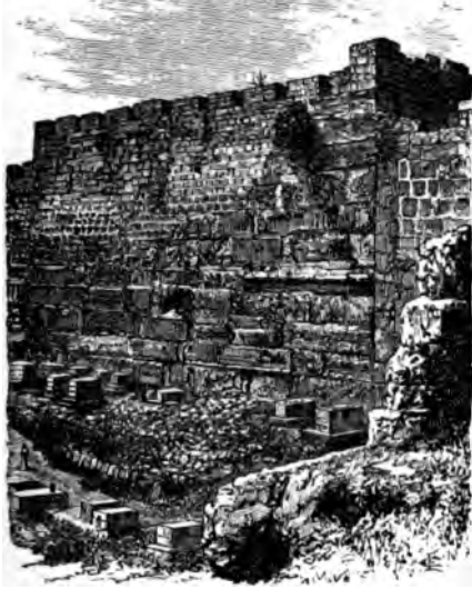
Foundation Stones on the Temple Area.
