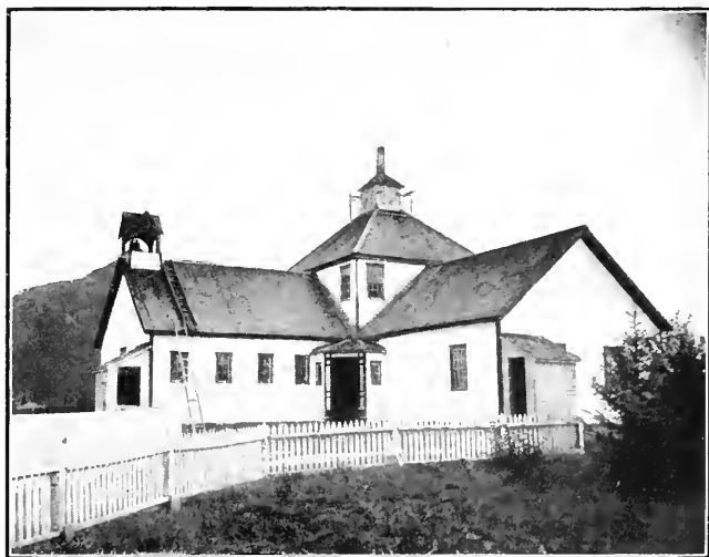
EDUCATIONAL BUILDING AT METLAKAHTLA
