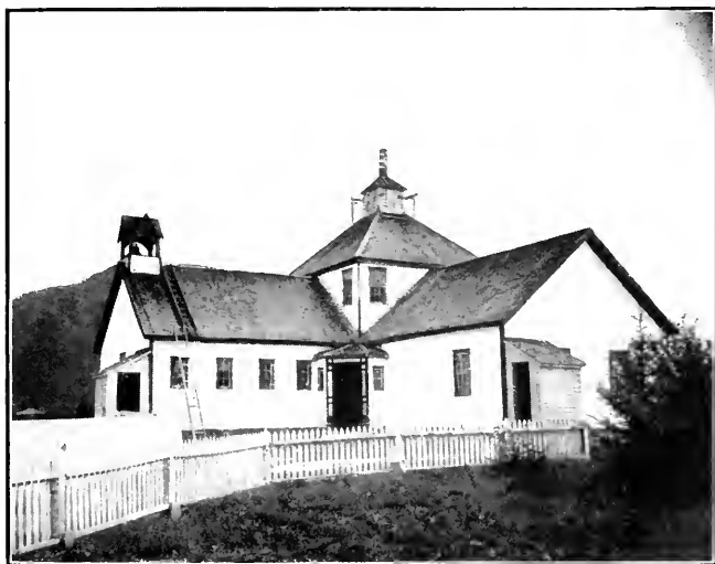
EDUCATIONAL BUILDING AT METLAKAHTLA
